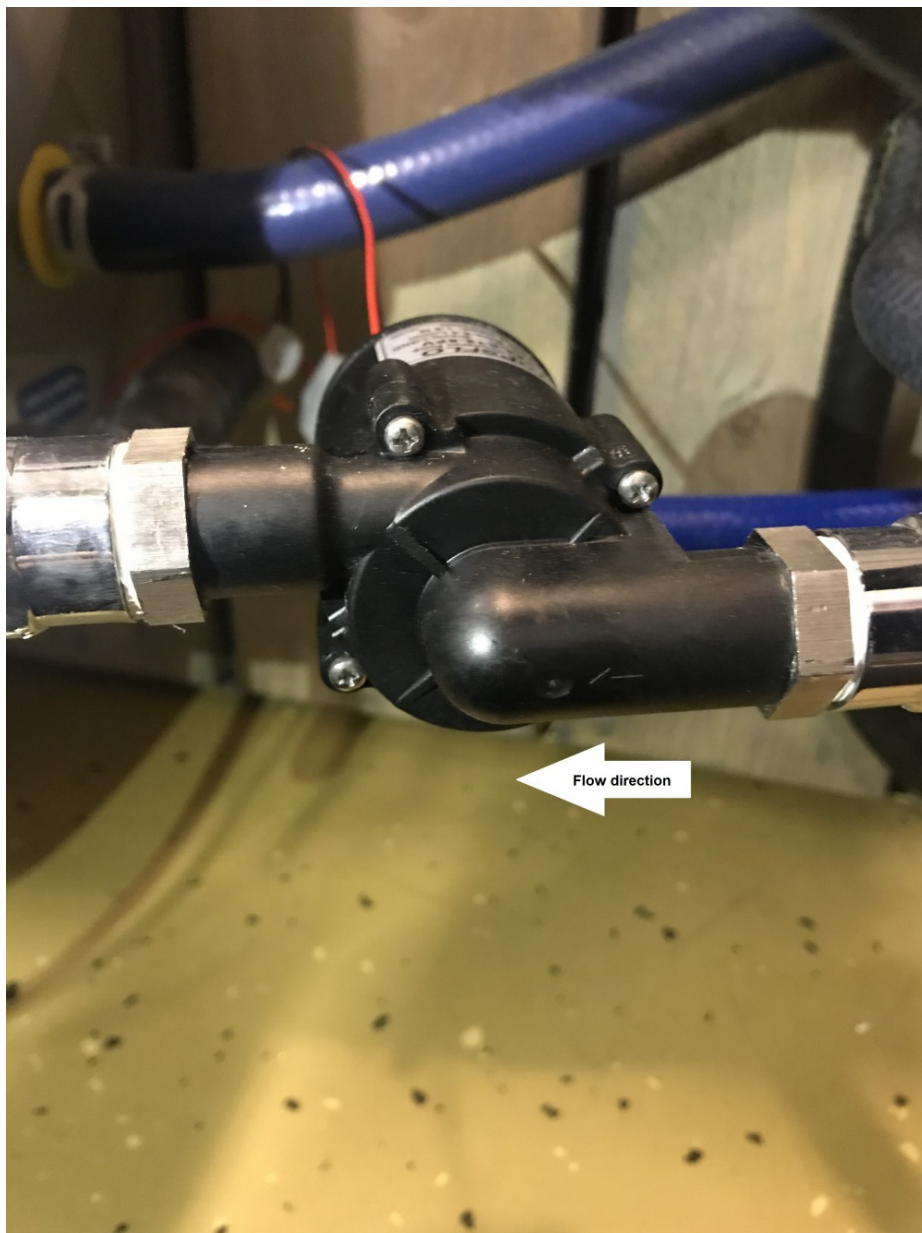
Arrow printed to the side of pump indicates flow direction.
